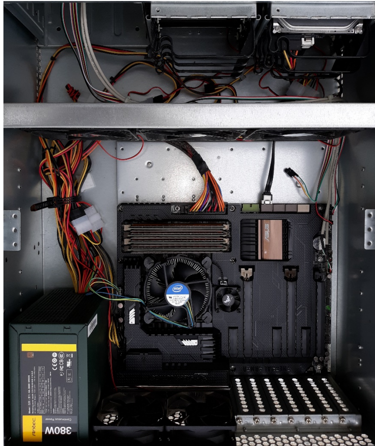
Figure 81 – View of the Inside of a Compute Node Chassis
